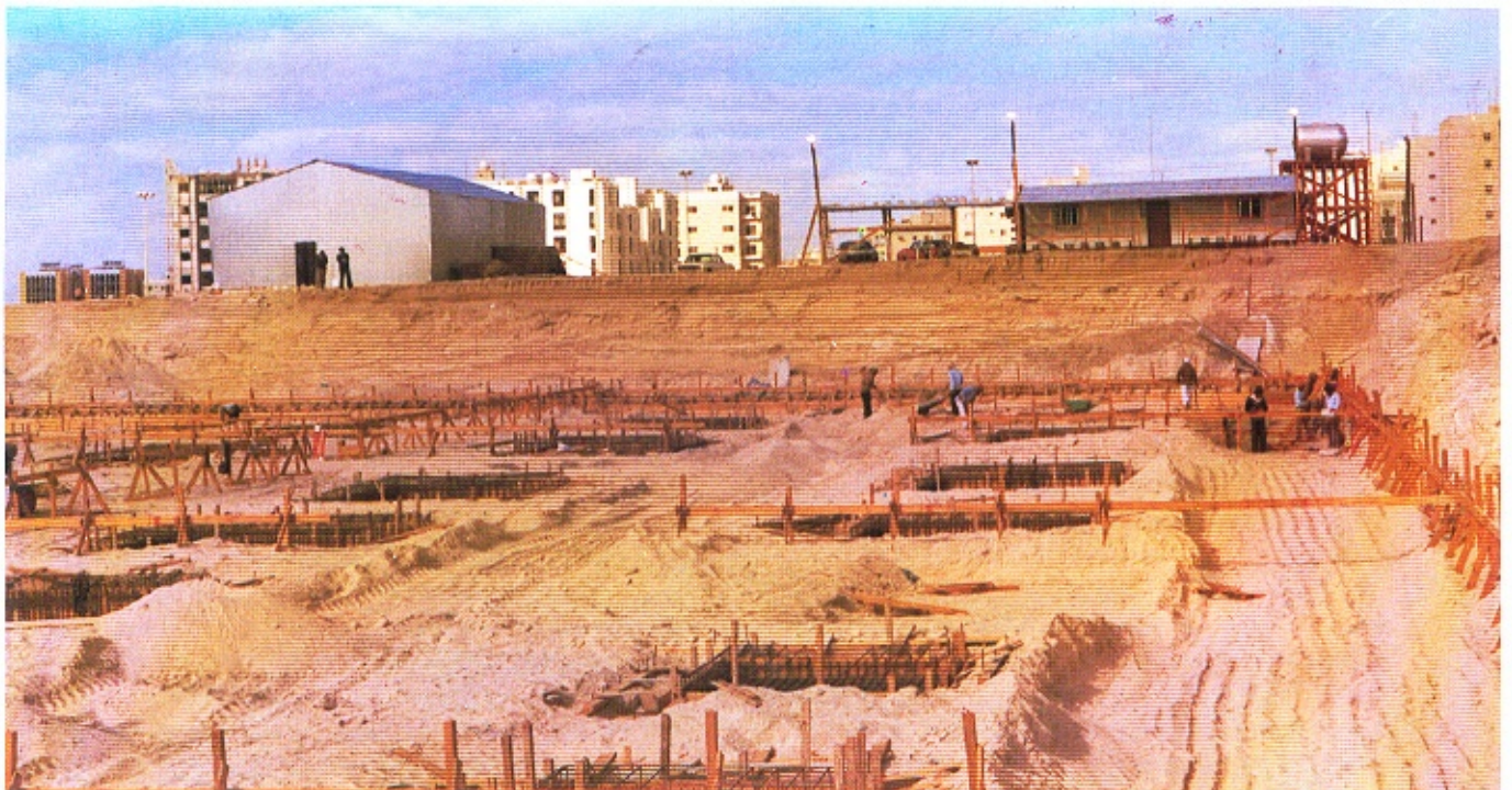
A project under construction - Construction Department
