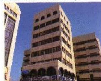
Building in Al-Hillah Street
